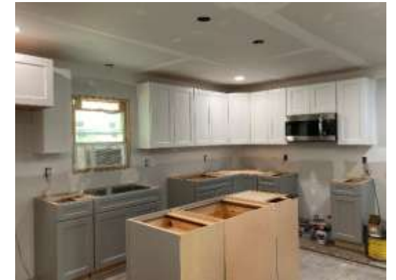
Renovations in Progress*
